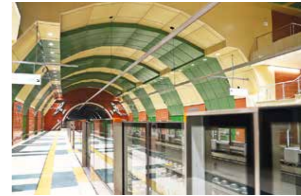
2020 / Metro Sofia - stanice Lvov most
